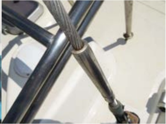
No corrosion at entry to swage terminals
