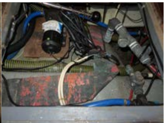
No sign of leak from pump
