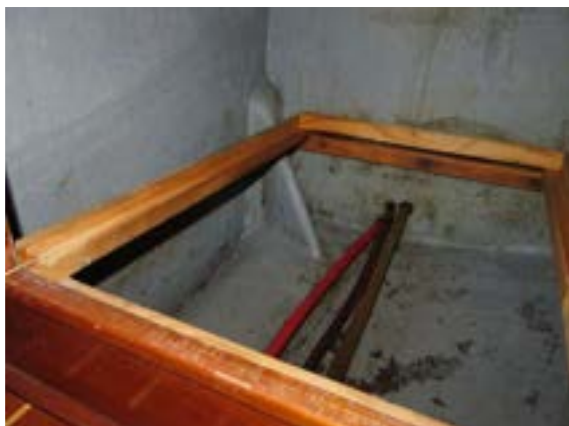
Intact bilge structure
