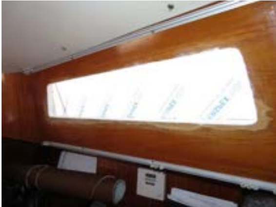
Side windows renewed
