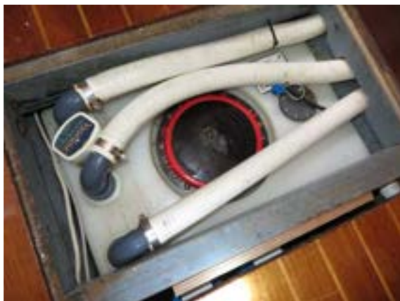
Black water tank externally intact
