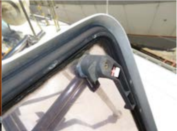
Hatch window seals not deteriorated
