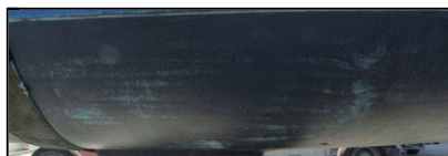
1.6 Item 2(Picture) Port Midship hull below W/L
