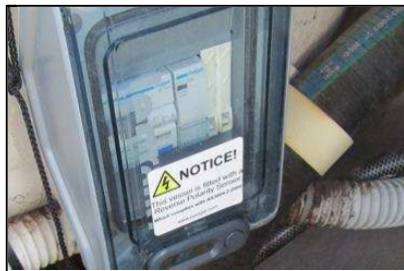
8.1 Item 1(Picture) Shore Power board 240 V AC
