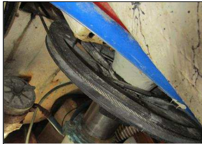
7.0 Item 1(Picture) Steering Gear Quadrant
