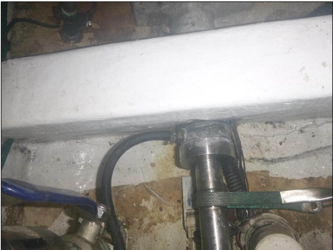
Starboard Shaft Seal
