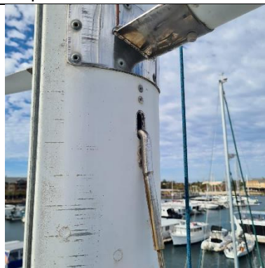
Spreader base attachment in good condition with minimum signs of corrosion.
